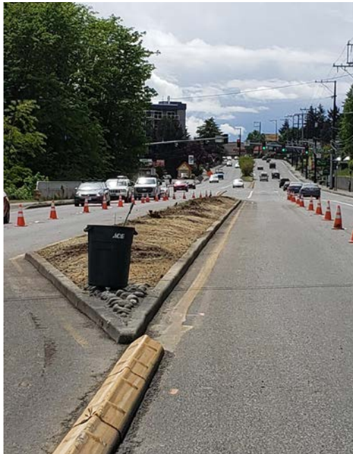
Public Works cleaned the center medians on SR-522.
