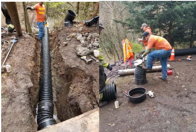
Drainage repair work in 3700 block of NE 205 th St.
