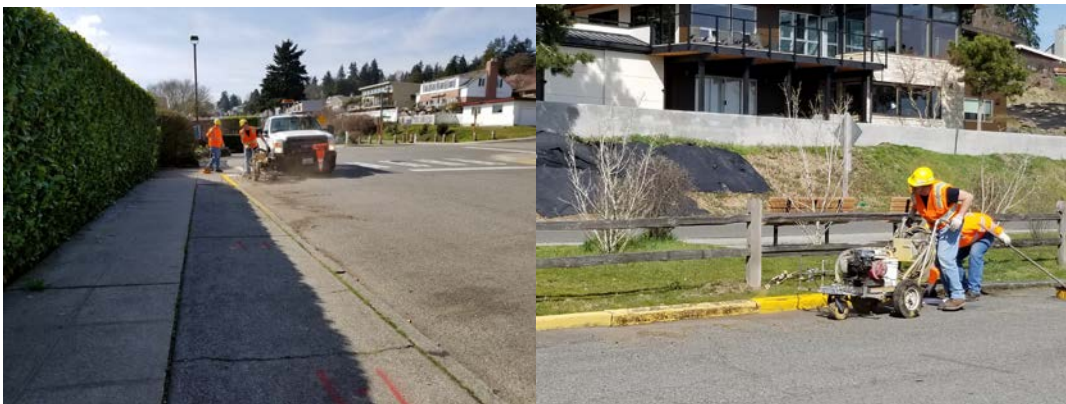
King County Traffic striping crews freshening up the Yellow paint on the No Parking areas on Beach Dr. NE near NE 165 th St.
