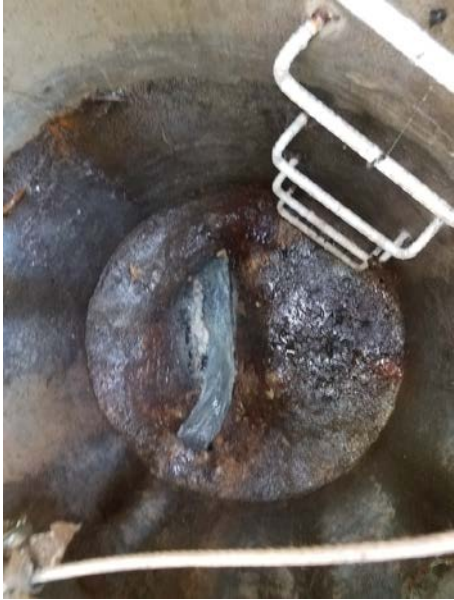
Sanitary sewer access portal inspections continue throughout the system.
