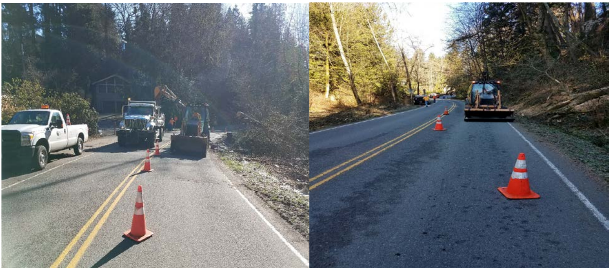
Public Works crew cleaning up fallen tree debris on Perkins Way.
